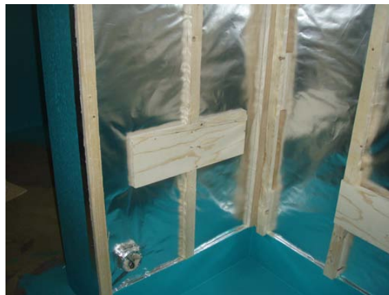
Figure 2. Vapor barrier and aluminum foil installation
