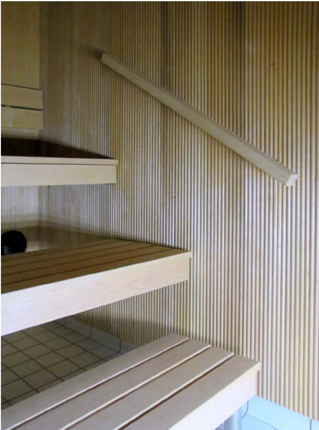
Figure 7. Yard sauna timber frame wall
