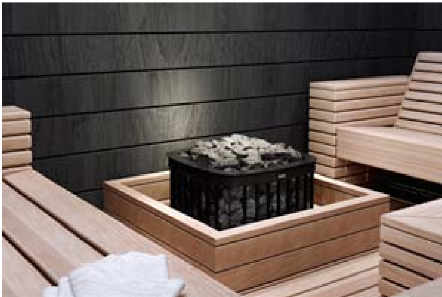
Safety clearance and protection installation
